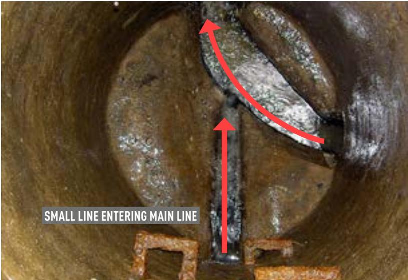
Converging sewer lines (as seen from the top of a manhole)
