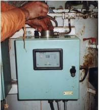
35, 36, 37. Example of 15ppm sensor and alarm. The pictures on the right show the testing of the alarm by unscrewing the plug and placing an object inside to block the light so that the equipment goes into alarm mode and the stopping device operates. Note that manufacturers of this equipment do not recommend placing hard objects down the sample tube. The test does not prove that the device is accurately calibrated.
