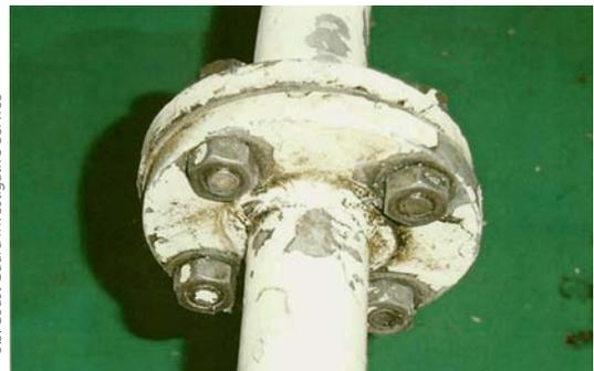
20. Evidence of chipped paint and worn bolts.
