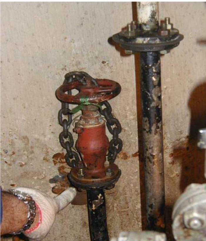
19. Evidence of repeated dismantling of piping connected to ODV. Note that the use of a chain and padlock does not prevent illegal discharges. It just means it is less likely for them to be accidental.
