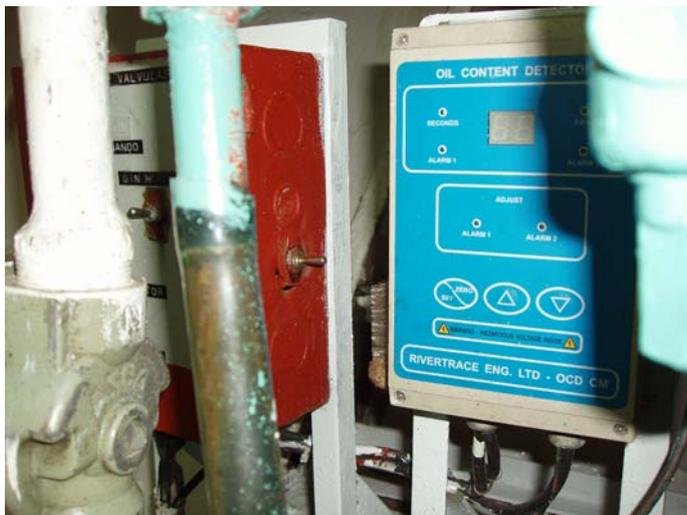
21. Bypass switch installed to silence the Oil Content Monitor alarm and allow the Oily Water Separator to continue to operate even when oil content is more than 15 ppm.
