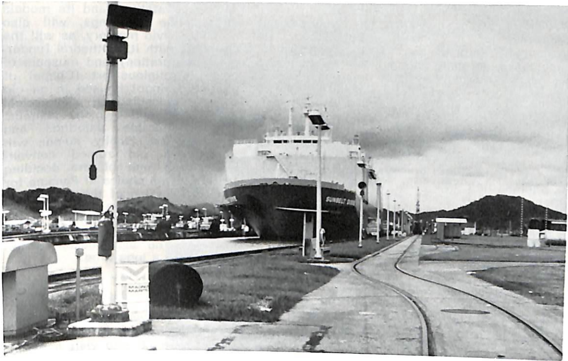
Panama Canal, Miraflores lock
