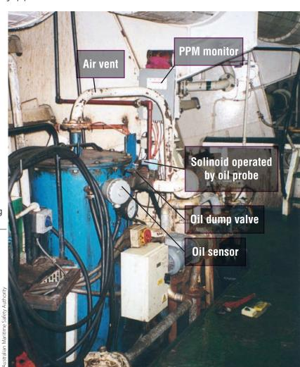
34. Another example of oil filtering equipment onboard a vessel.
