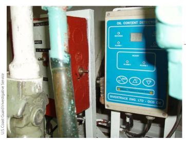
21. Bypass switch installed to silence the Oil Content Monitor alarm and allow the Oily Water Separator to continue to operate even when oil content is more than 15 ppm.
