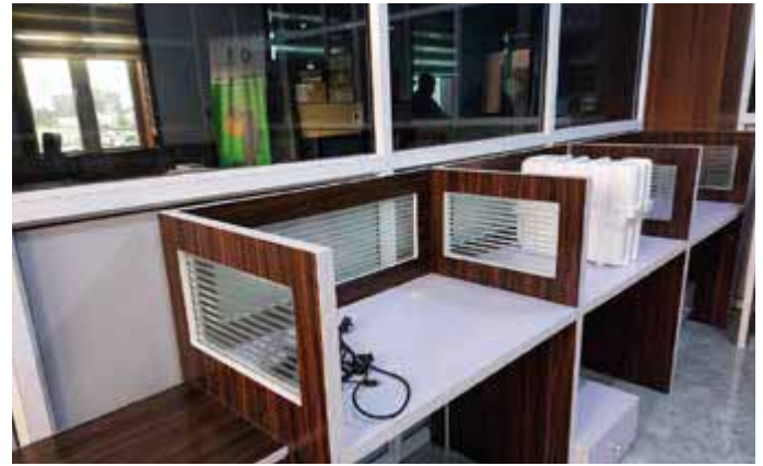
Renovation work on the future DACORE premises in Nigeria
